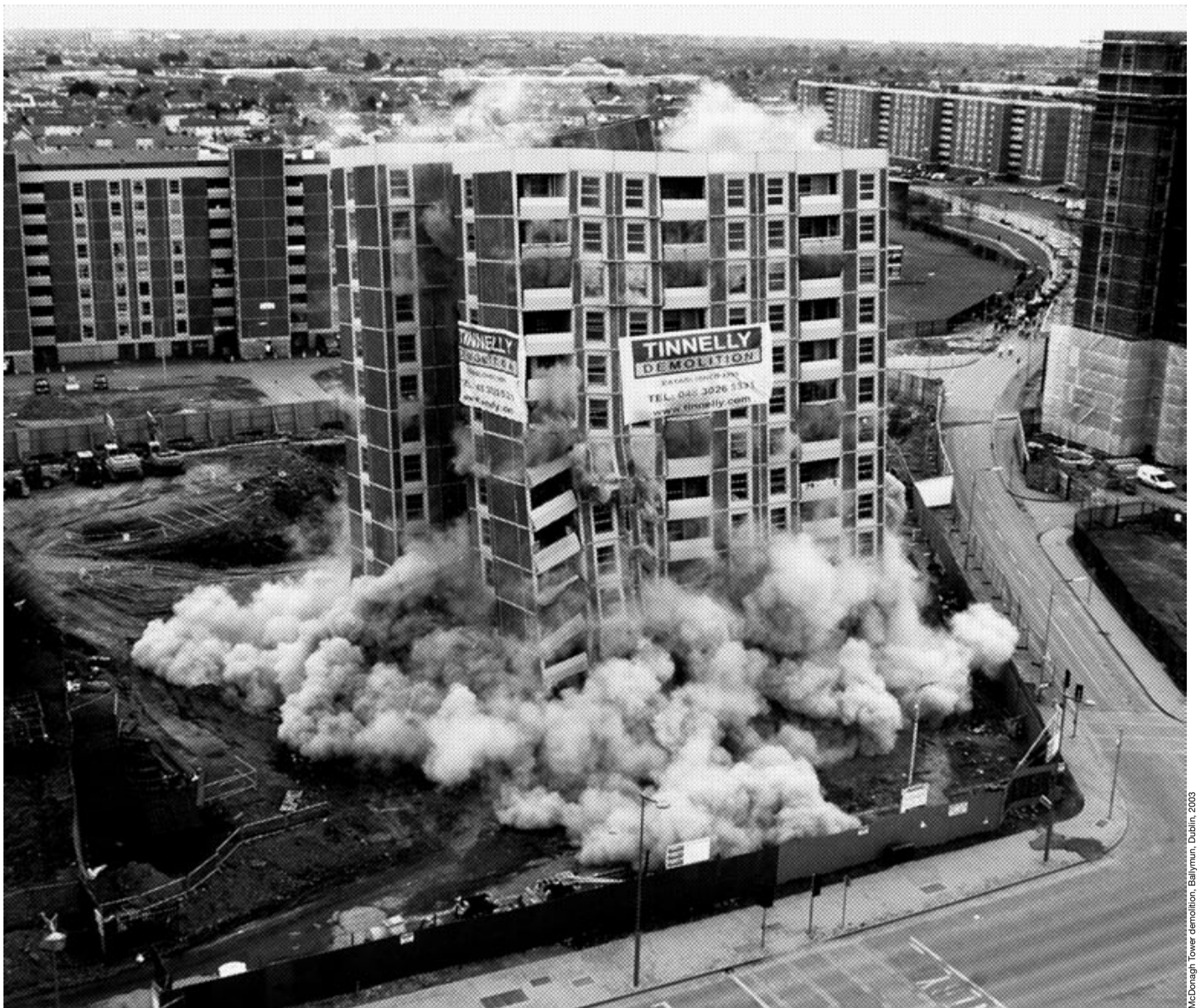
McDonagh Tower demolition, Ballymun, Dublin, 2003
